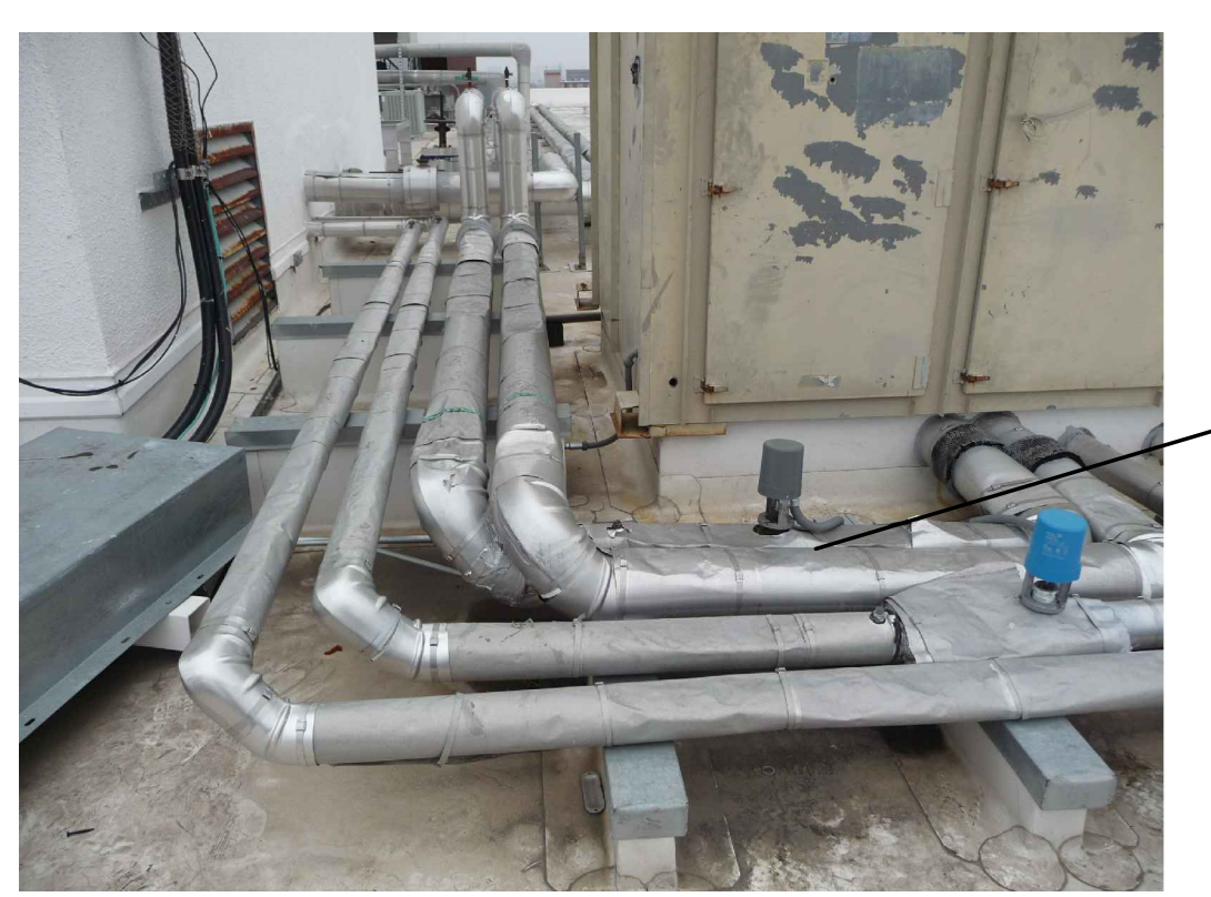
5 SW OAHU CHILLED AND HOT WATER PIPING
