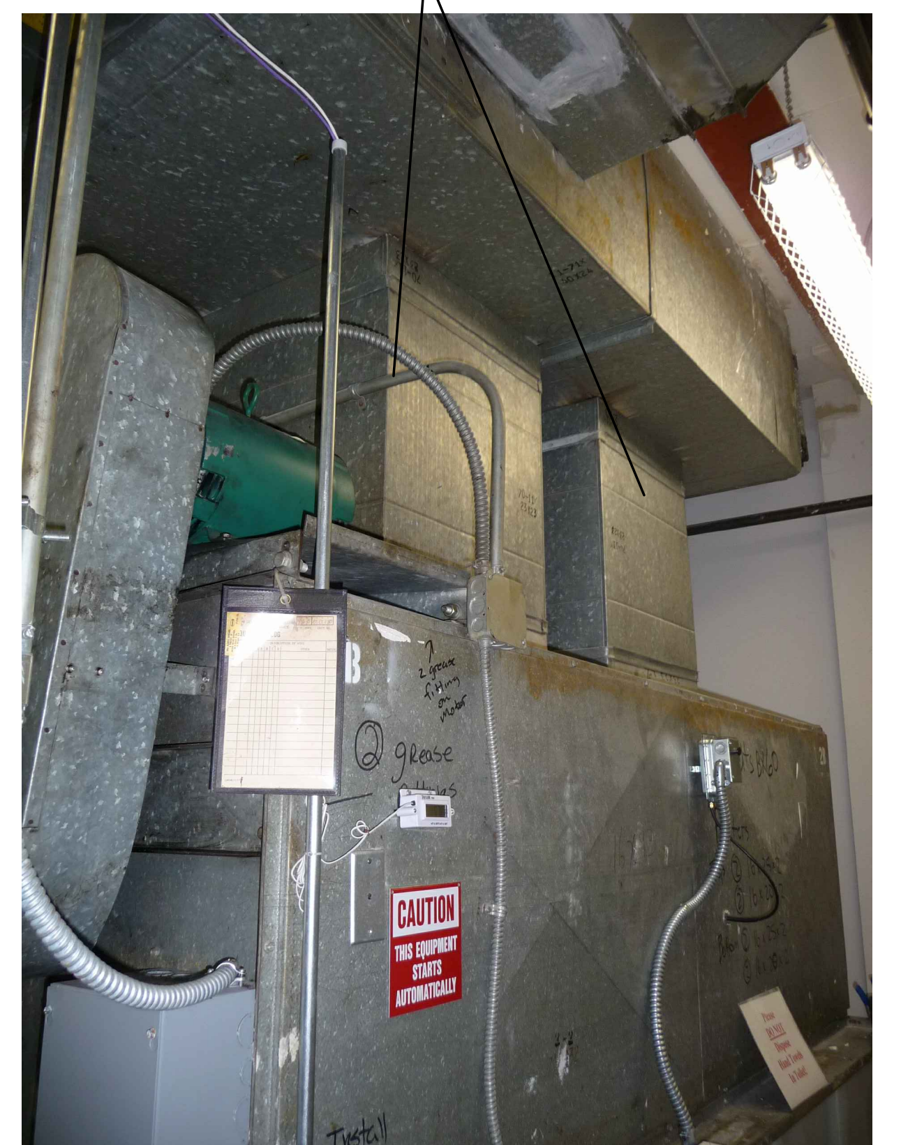
3 AHU-2-SW DUCT CONNECTIONS SCALE: NO SCALE
